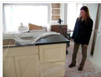
Natalie Lewis, owner of Got Green Goods?, shows off the home's new shetkaSTONE countertops that are made from recycled paper. Photo by Sam Calhoun
