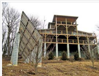
The 3.69-kilowatt solar power system will produce about $70 worth of energy credit every month for the Gaul family in Blowing Rock. The power produced from the system will be fed back into the BREMCO grid, and the homeowners will receive a payment for the power quarterly. Photo by Sam Calhoun
